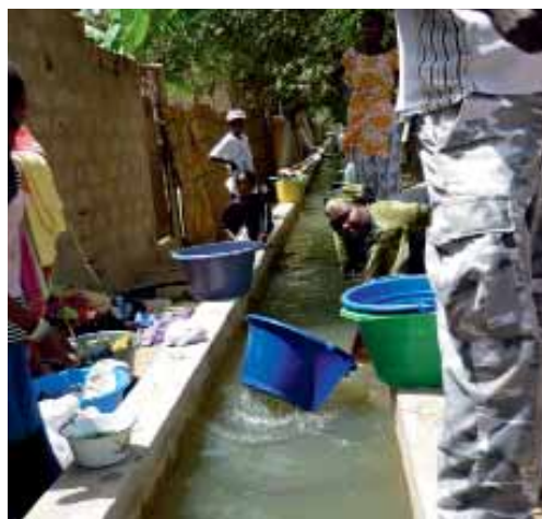
Aqueducts transport water in Saint Louis, Senegal © UN-Habitat/Marie Dariel-Scognamillo
