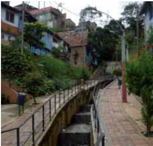
Drainage infrastructure greatly improves the conditions of sloping areas in Medellin, Colombia © UN-Habitat/Laura Petrella
