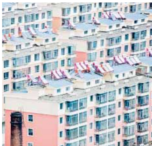
Solar water heating in Hunchun, China © UN-Habitat/Alessandro Scotti
