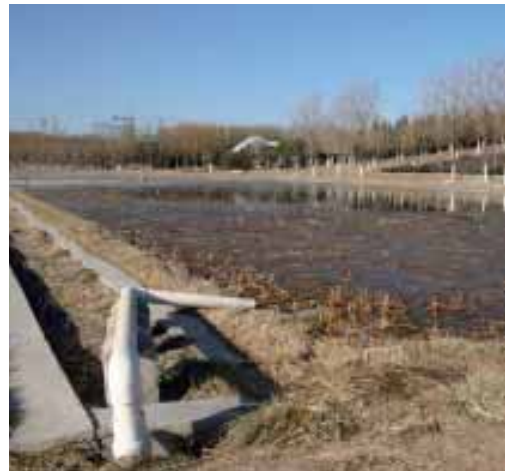
Constructed wetland in Olympic Forest Park, Beijing, China © Flickr/Sustainable sanitation
