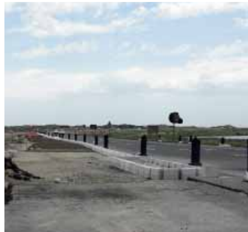
Road under construction, Cape Town, South Africa © Flickr/Warrenski
